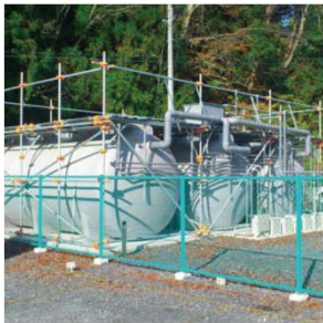
Example of a temporary housing installation following Japan's "Great East Earthquake" of 2011
