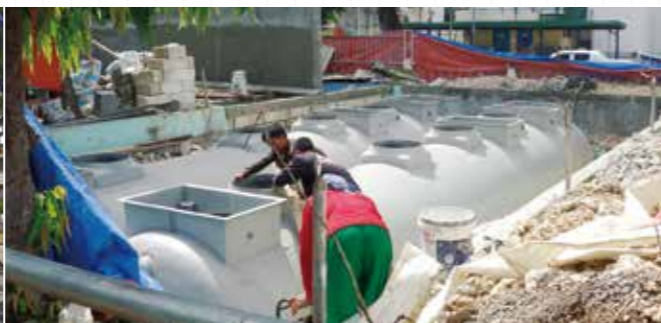
設置工事の様子 Scene from installation work
