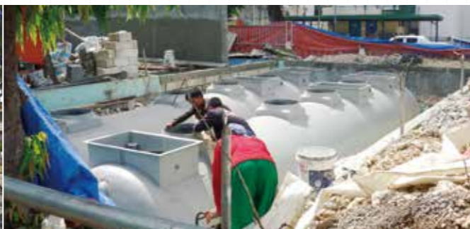
設置工事の様子 Scene from installation work
